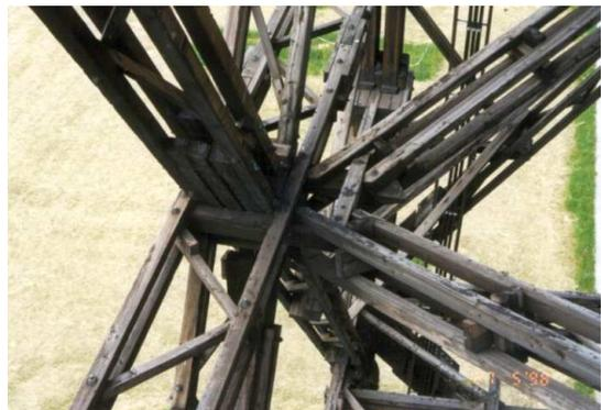
FIG. 9. View of the joint of diagonals, purlins and the spatial bracing (photo: A. Malczyk 1998) [2].
